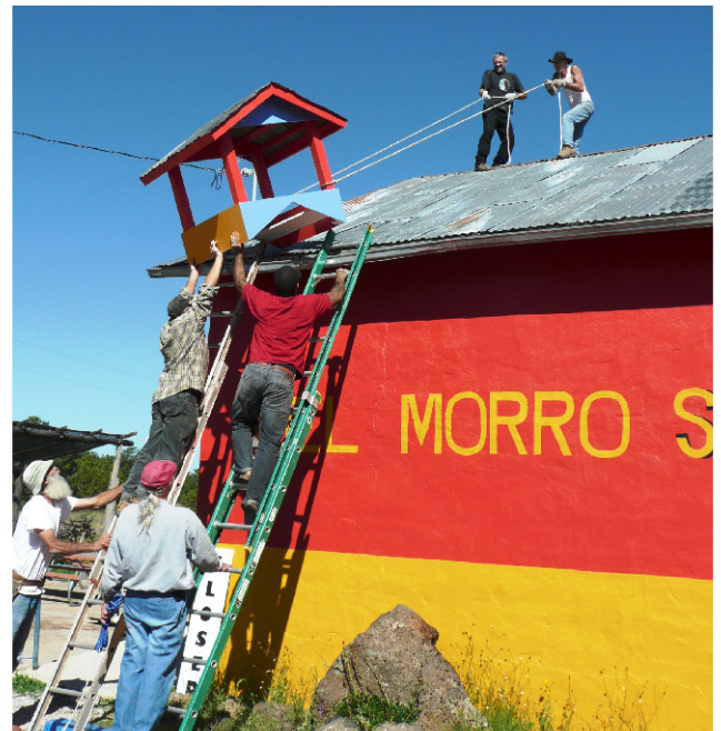
The Bell Tower goes up on newly-painted Old School Gallery.
